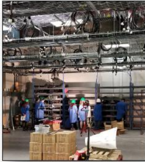
Initial infrastructure build out phase
